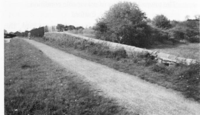
Site of Little Cut Junction in 2012. Photo Ken Geddes
